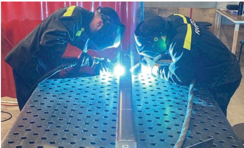
Figure 40. Boom structure welding.
